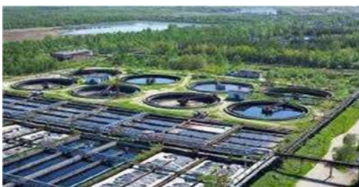
Fig 87: urban sewage treatment plant
