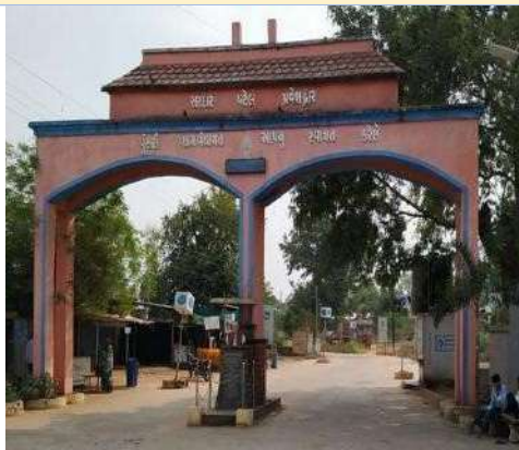
FIG.7: ENTRANCE GATE PUNSARI
